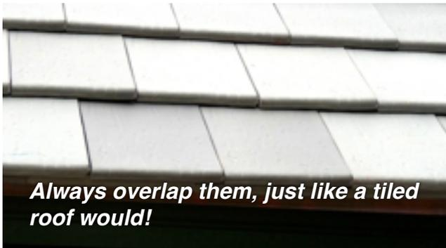
Keep repeating this step as you move **UP** the roof towards its peak, but always **remember**: You want the following layer to hang just over the last one so its like roofing tiles. Any part that has a chimney (or other obstruction), you merely cut pieces to go around the structure as shown. Make sure you keep the same number of rows.
